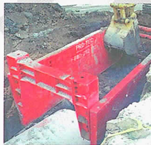
High Clearance Arch
